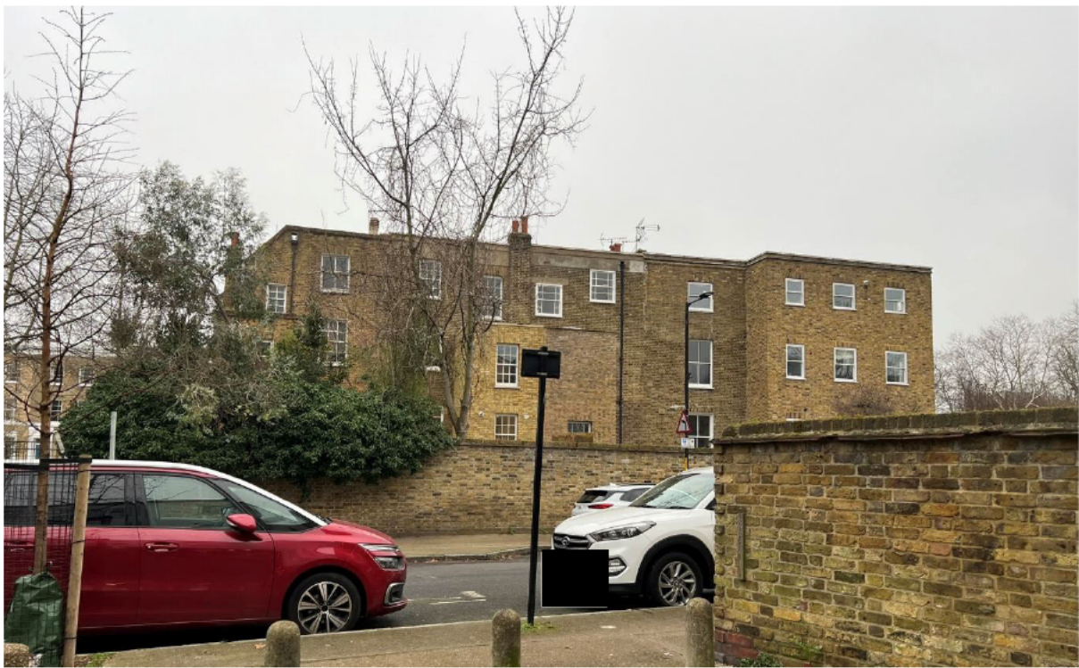
Rear of nos. 30-33 Sutherland Square (grade II listed)
