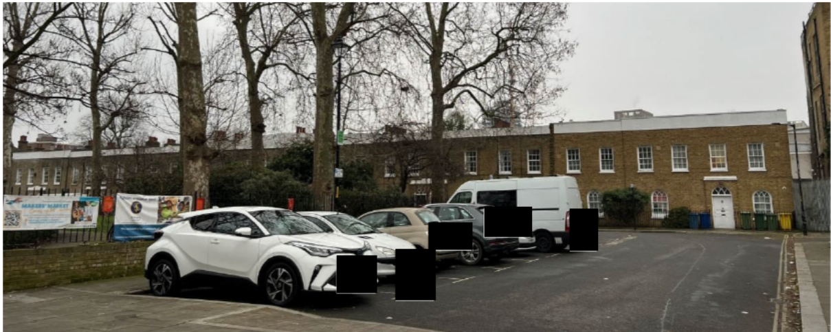
Nos. 28-52 (even) Liverpool Grove (grade II listed).
