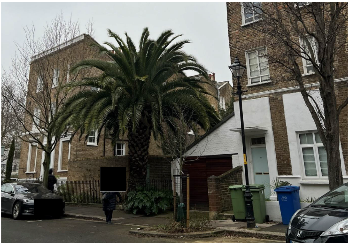
Butterfly roof to nos. 58-60 Sutherland Square (grade II listed), somewhat visible from the rear.
