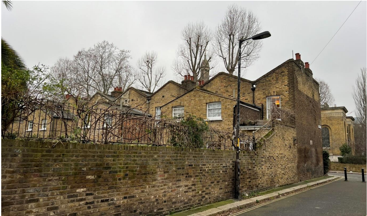
Butterfly roof of nos. 42-52 (even) Liverpool Grove, visible from the rear.
