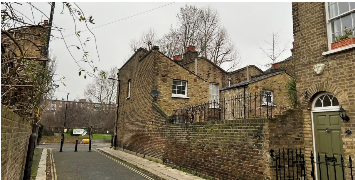
Butterfly roof of nos. 52-58 (even) Liverpool Grove, visible from the rear.
