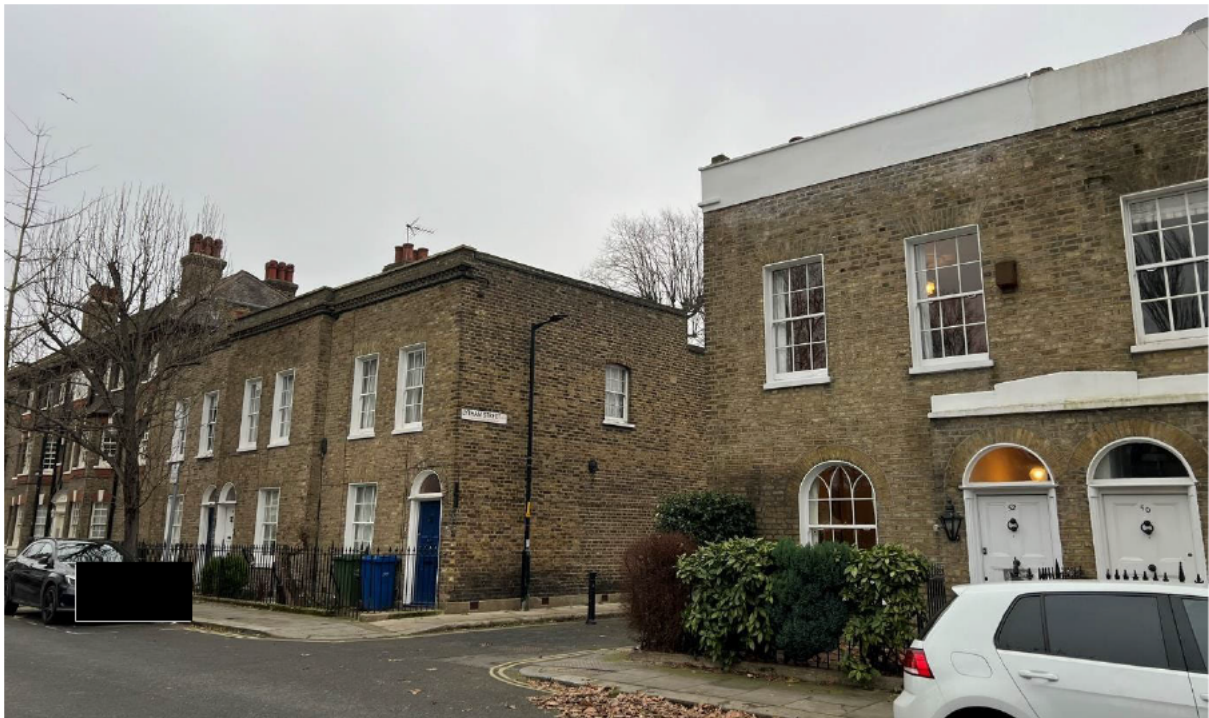
Nos. 50-58 (even) Liverpool Grove (grade II listed).
