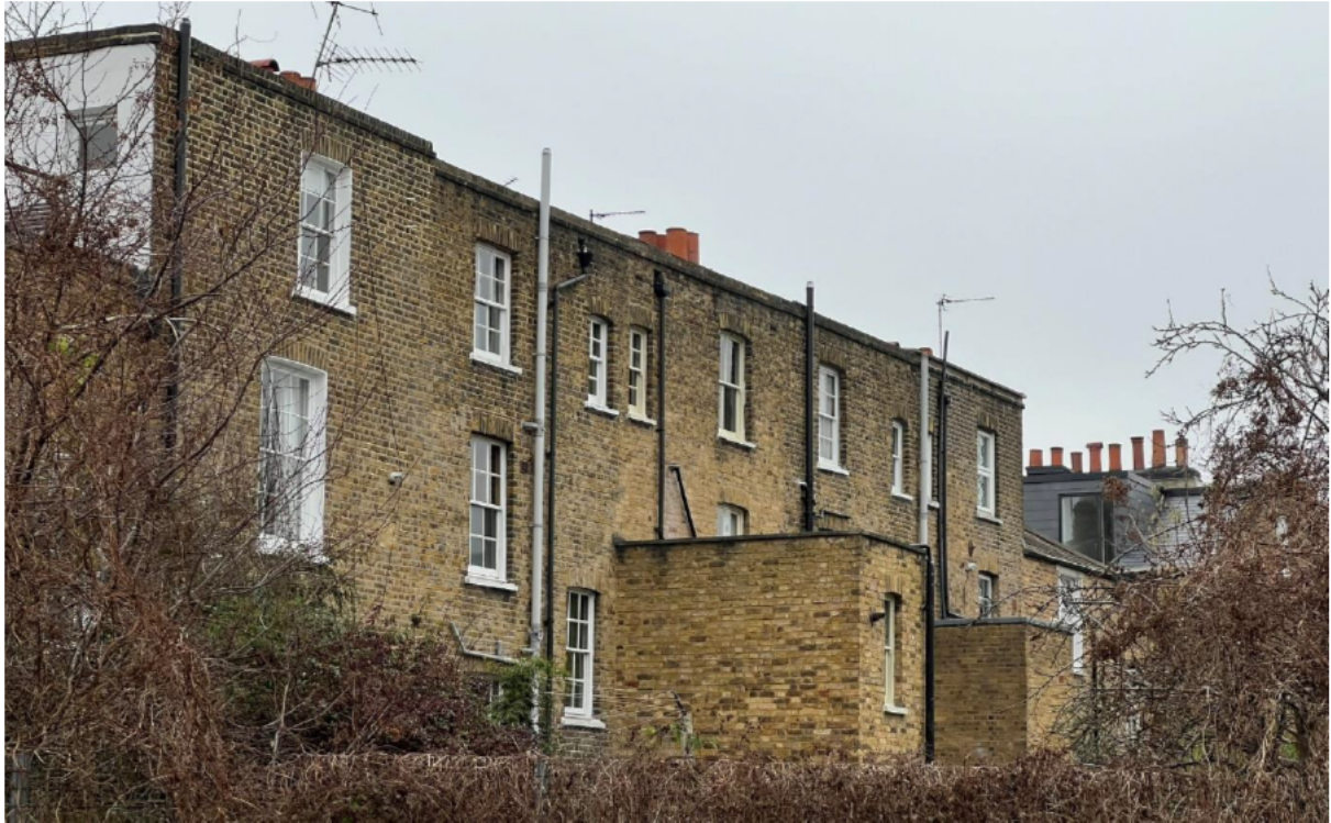
Rear of nos. 24-29 Sutherland Square (grade II listed).
